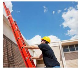
Your ladder material is important. Fiberglass ladders are sturdy, non-corrosive, and non-conductive if clean and dry, so use them for working around electricity. Aluminum ladders are lightweight and durable, but should NOT be used around electricity.
